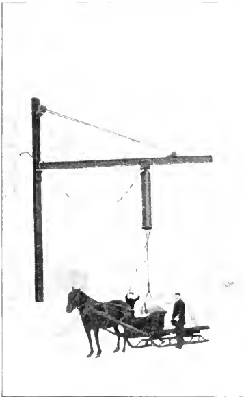
Jib Crane mounted on outside wall of building for loading and unloading material
